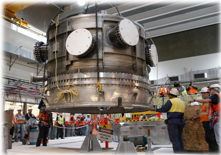
Figure 2: OPAL heavy water tank [3]
